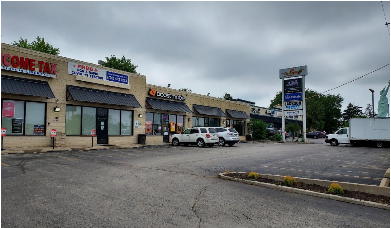
Figure 1: Five-unit commercial building at 224 – 232 S. Larkin Avenue
