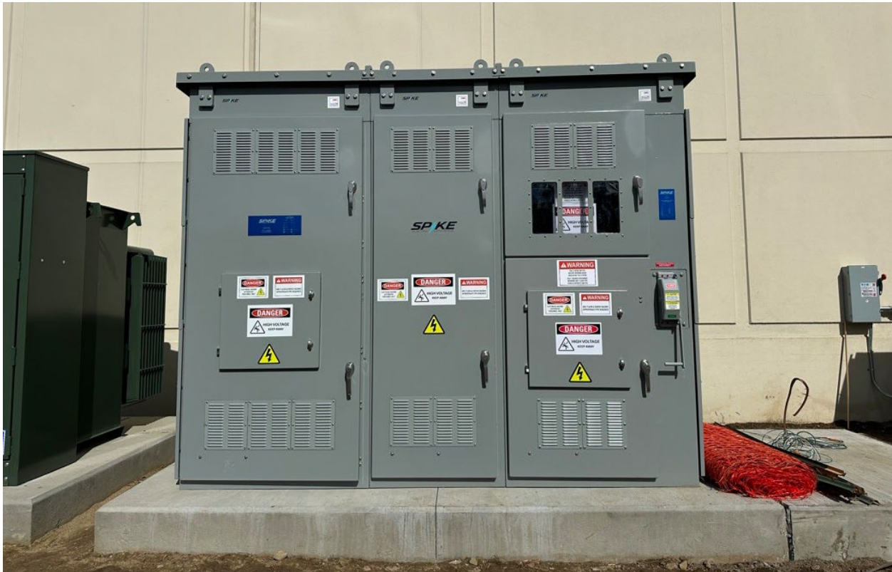
Figure 4: Equipment example: MV Disconnect
