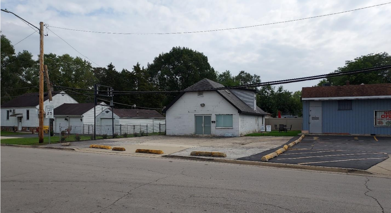
Figure 1: 102 Doris Avenue, view south from Doris Avenue near Gardner Street intersection
