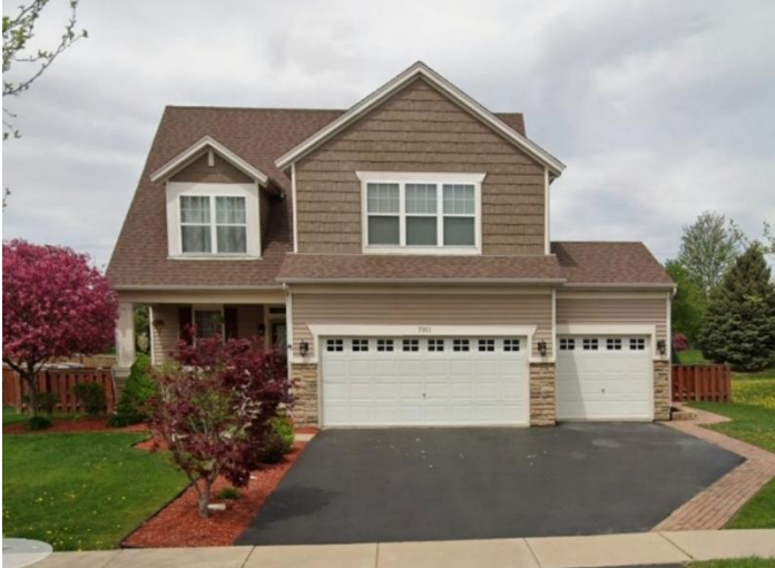
Figure 6: Existing residences in NeuStoneshire Phase One (2023, 2025)
