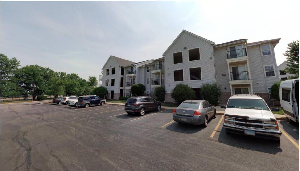
Figure 2: Existing residential building at the subject site (June 2023)
