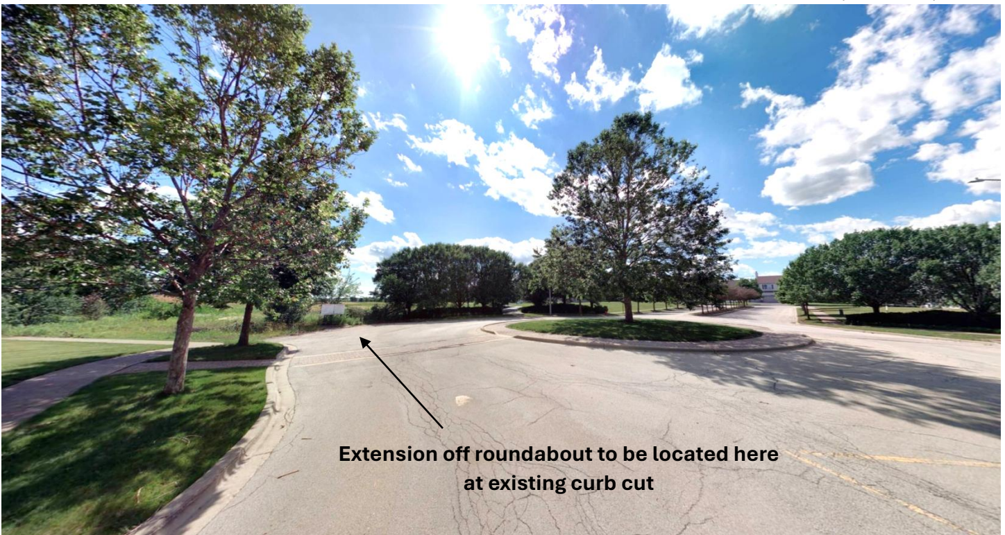
Figure 6: Existing roundabout for Neustoneshire Boulevard off County Line Road, view southwest (June 2026)
