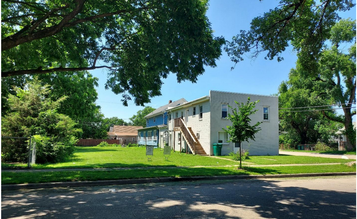
Figure 2: Subject site at 303 S. Ottawa Street (where signs are posted), and adjacent lot under common ownership at 301 S. Ottawa Street (blue and white buildings), view west from Ottawa Street (July 2026)
