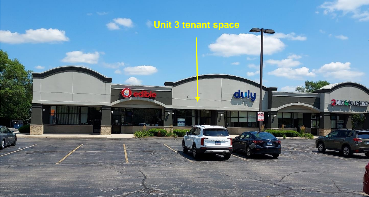
Figure 3: Unit 3 in 1504 Essington Road building
