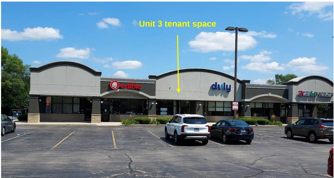
Figure 3: Unit 3 in 1504 Essington Road building
