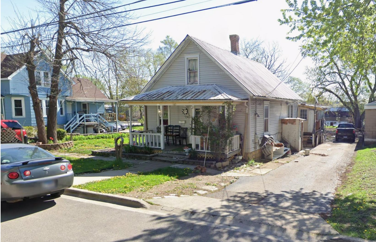
Figure 1: One-and-a-half-story structure at 540 Bluff Street (April 2025)
