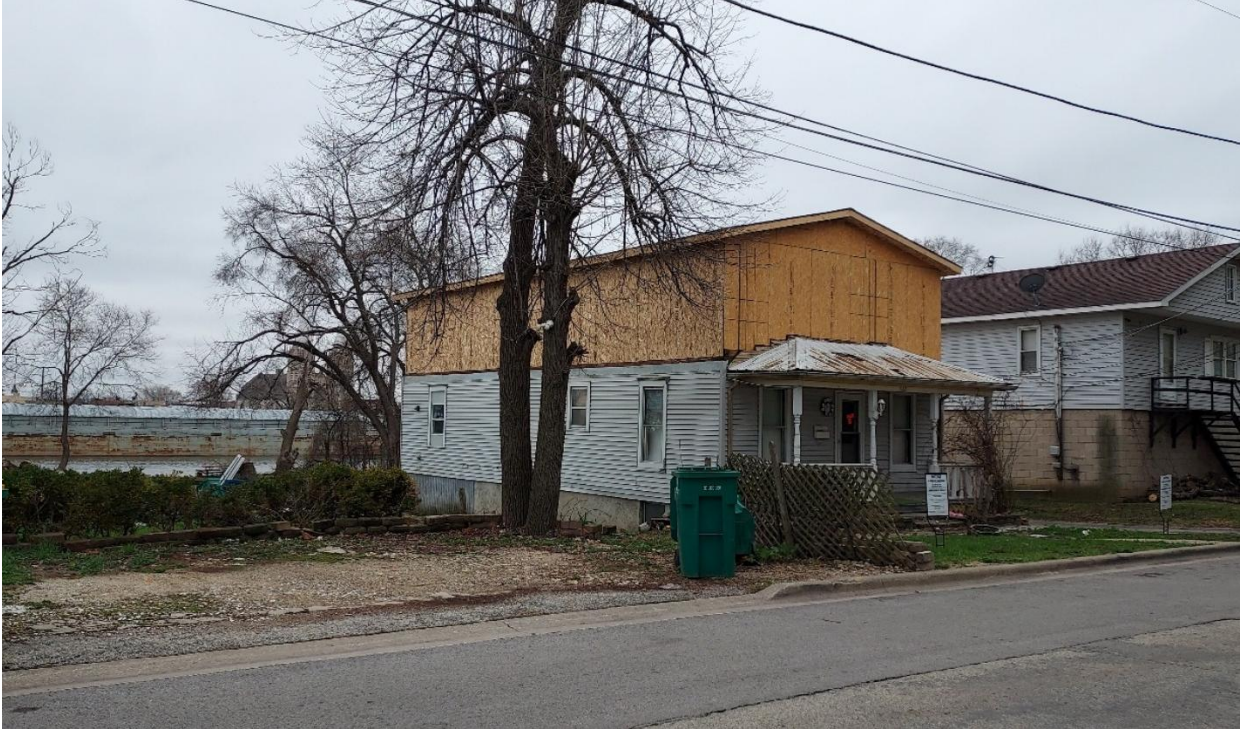
Figure 3: Current structure at 540 Bluff Street (April 2026)
