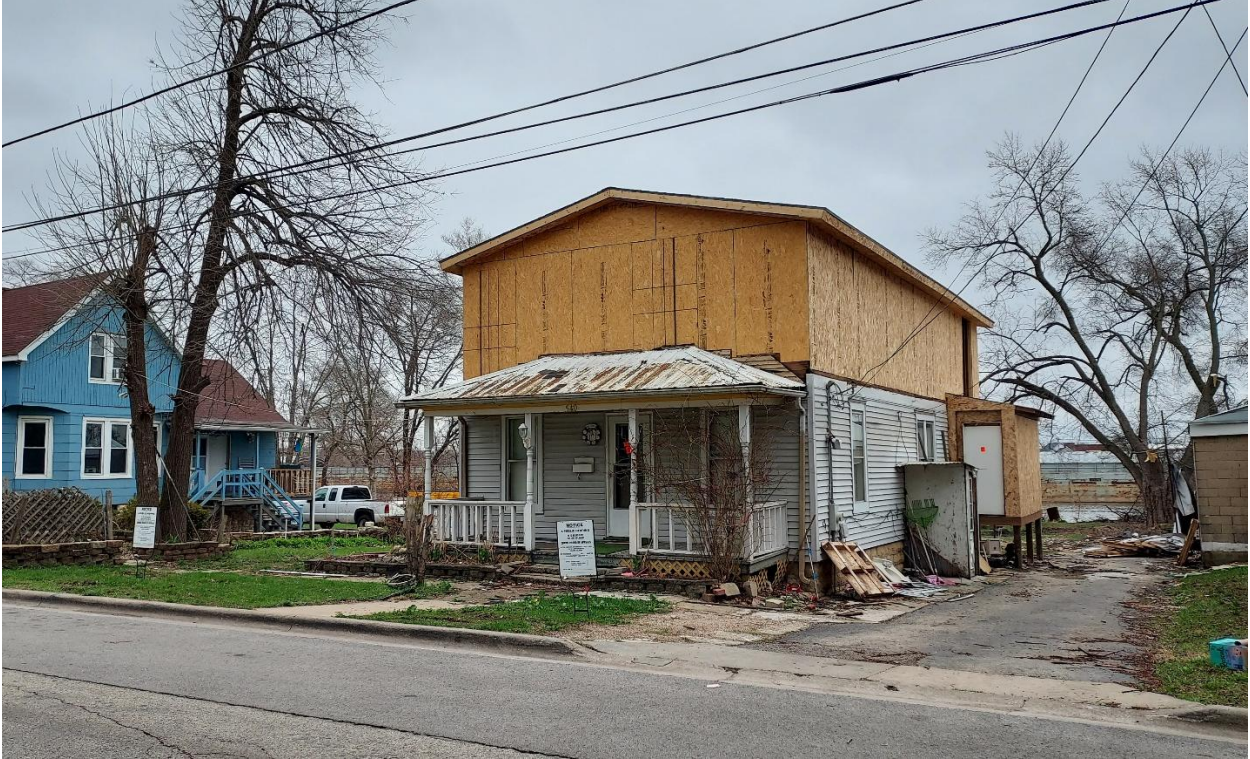
Figure 2: Current structure at 540 Bluff Street (April 2026)
