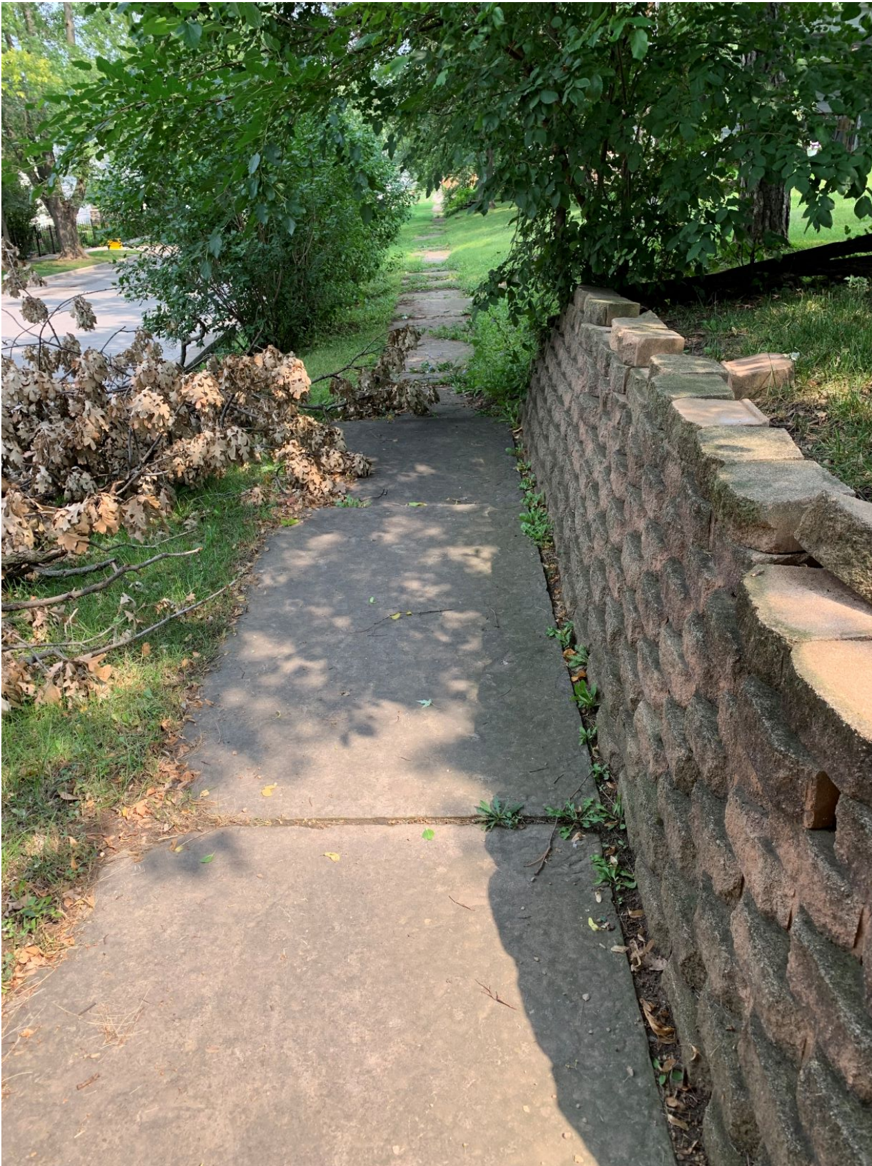
Figure 5: Front sidewalks (facing north)
