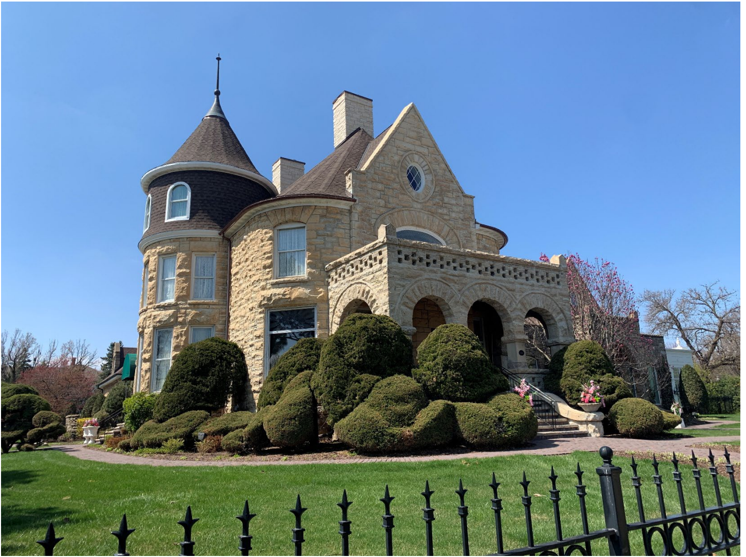
April 2025 after restoration work
