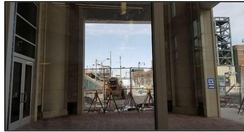
Gateway Transportation Center Under Construction
