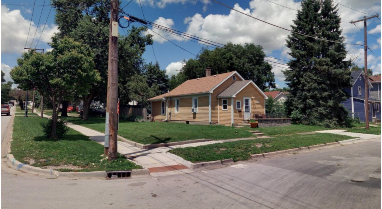
Figure 5: Existing residence at 329 Pleasant Street, view northwest from the intersection of McDonough Street and Pleasant Street (June 2026)
