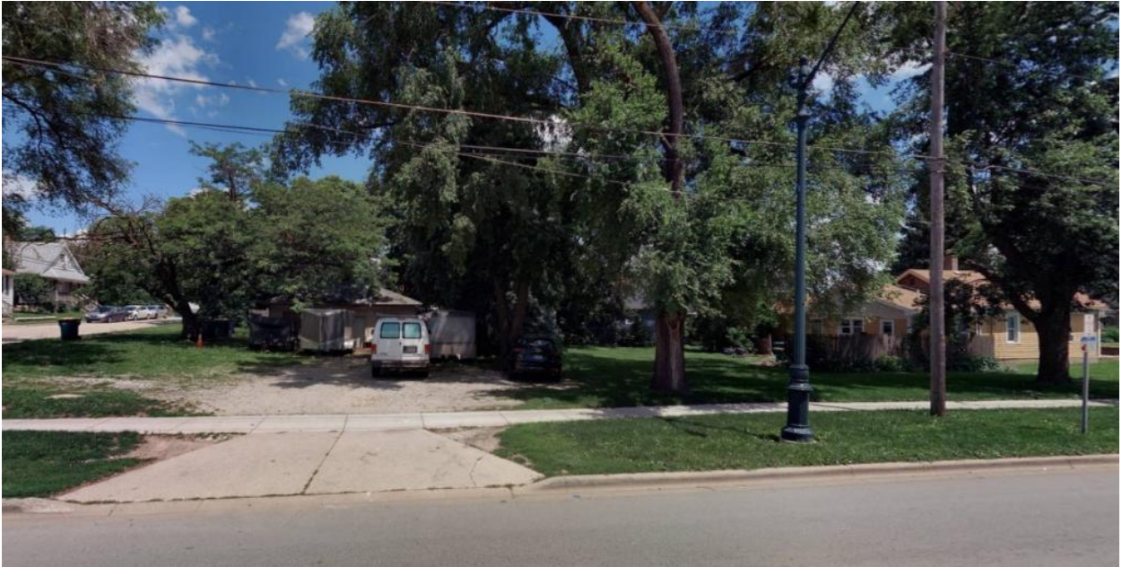
Figure 3: Subject site at 329 Pleasant Street, view north from McDonough Street (June 2026)
