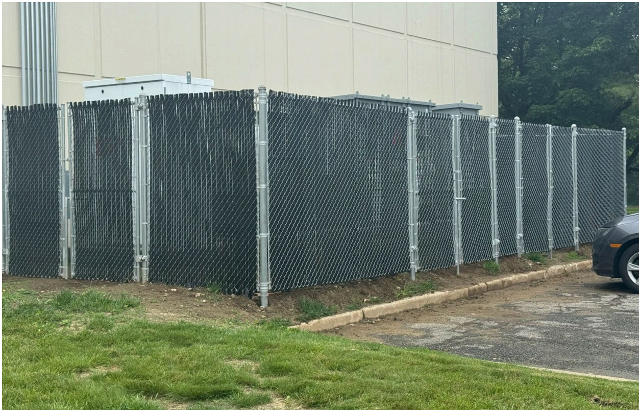
Figure 7: Building equipment enclosure example: chain-link fence with slats
