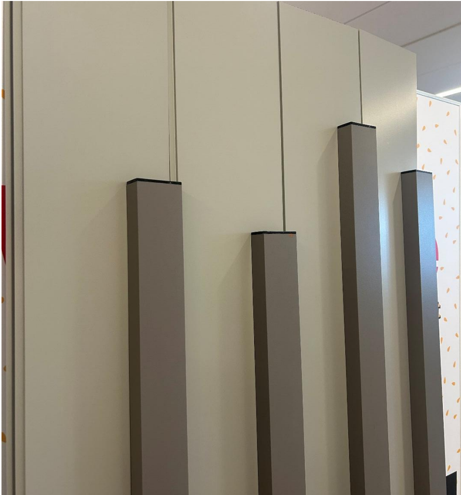
Figure 4: Sample of aluminum cladding with aluminum batten accents
