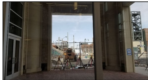
Gateway Transportation Center Under Construction
