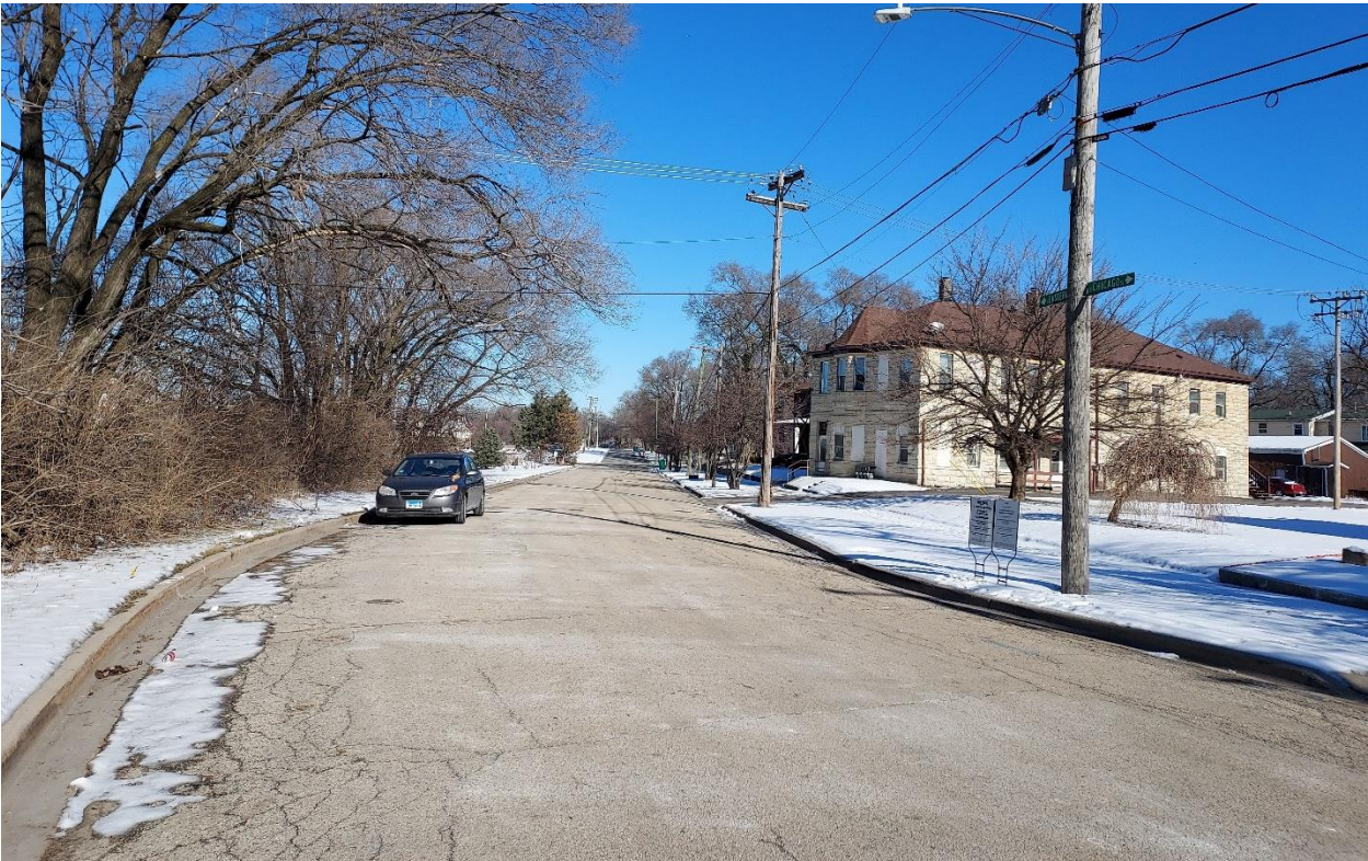
Figure 2: South Eastern Avenue, view north from South Chicago Street
