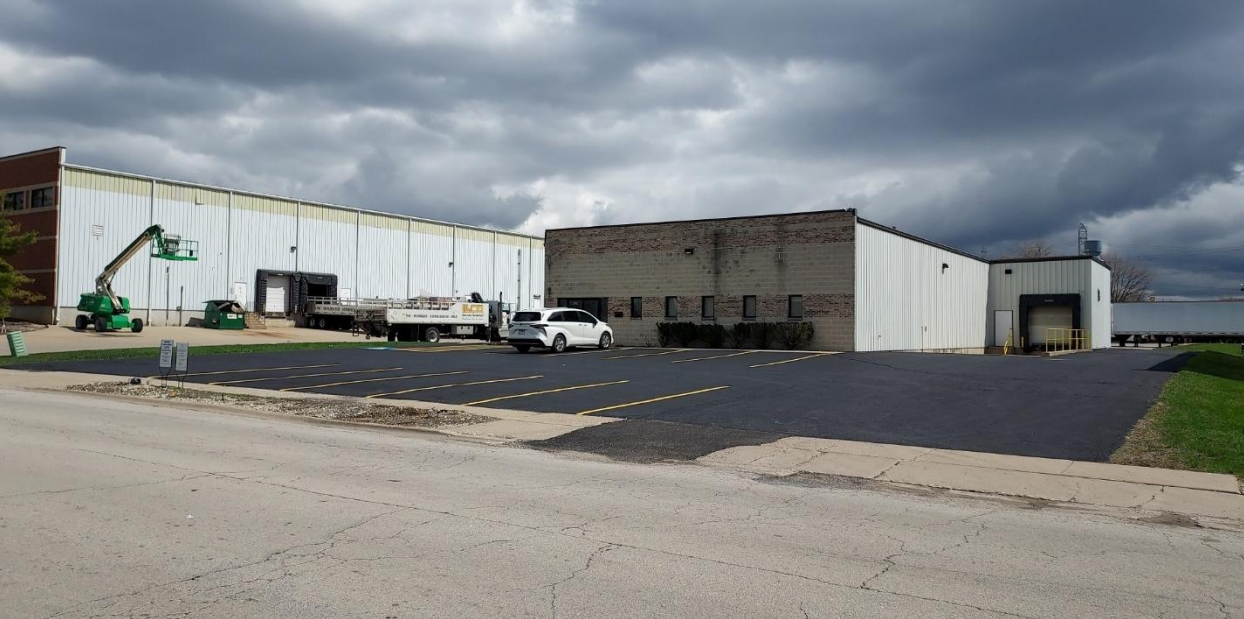
Figure 2: 470 S. Hammes Avenue, view northeast from Hammes Avenue (April 2025)
