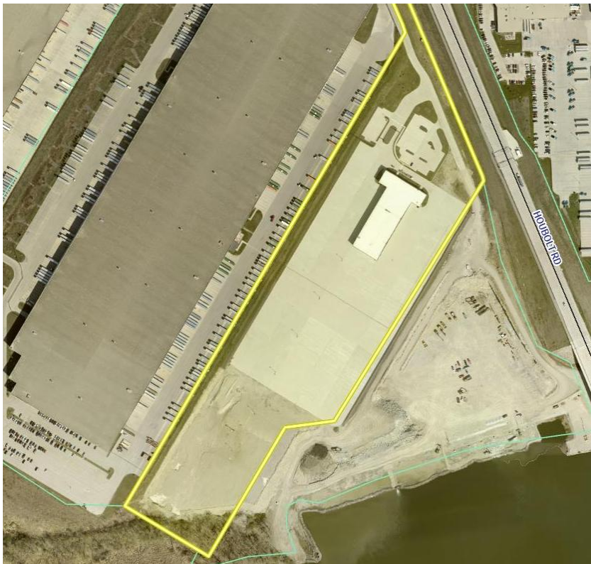
Figure 2: Existing building and paved parking area on the subject site (2025)
