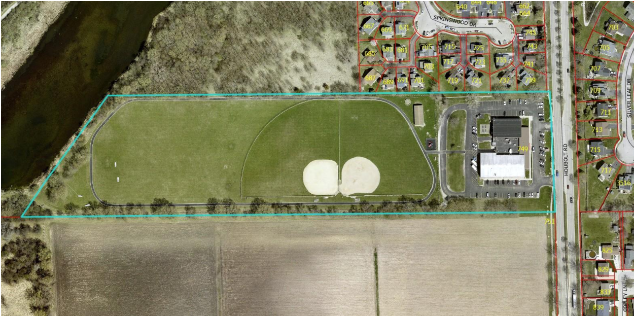
Figure 1: Aerial view of subject site at 749 Houbolt Road (2025)
