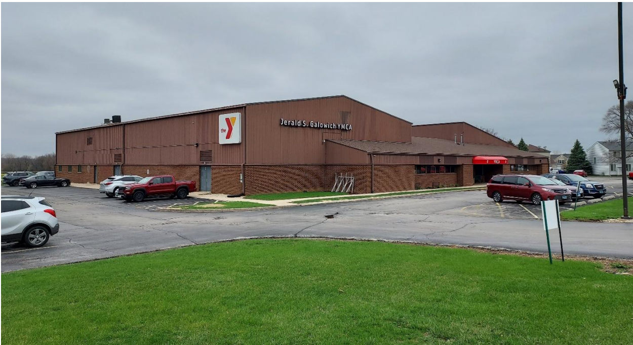
Figure 2: Existing building at 749 Houbolt Road, view northwest from Houbolt Road (April 2026)
