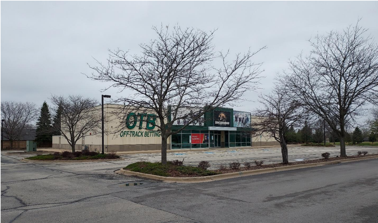
Figure 4: Existing building on subject site, view southwest from interior road along north of site (April 2026)
