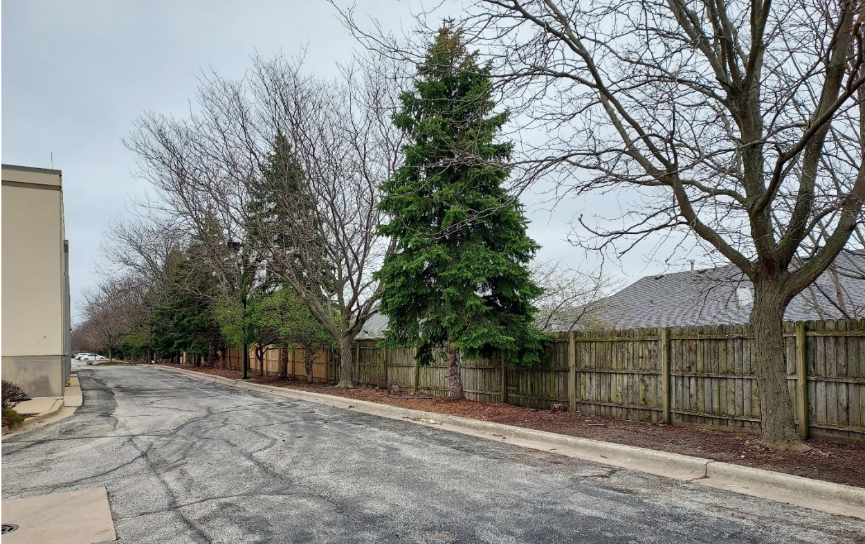
Figure 6: Existing landscape area and fence along south property line behind existing building, view looking southeast (April 2026)
