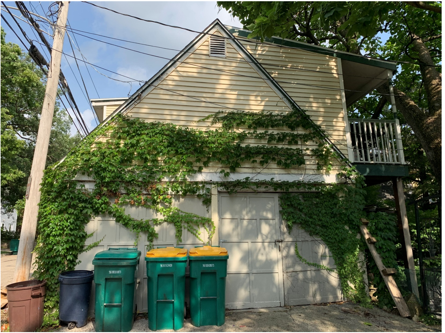
Figure 2: West elevation of the upper apartment unit
