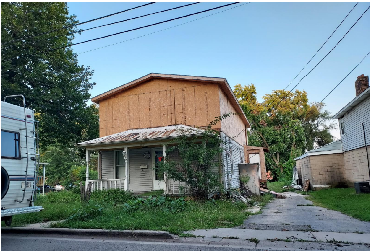
Figure 2: Current structure at 540 Bluff Street (August 2026)
