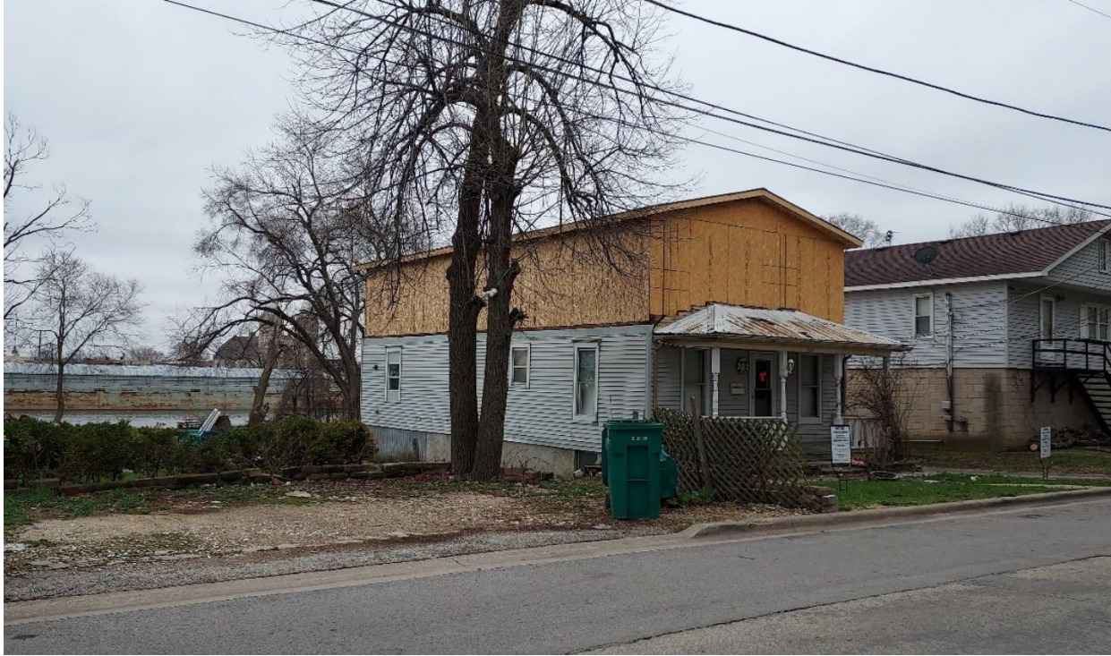
Figure 3: Current structure at 540 Bluff Street (April 2026)
