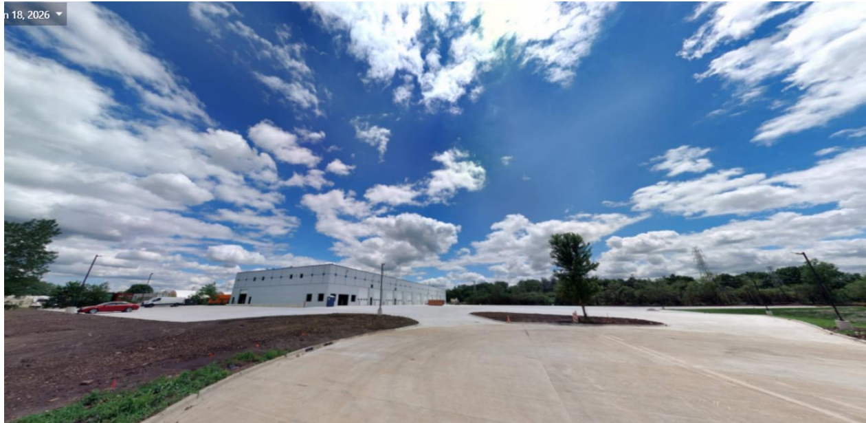
Figure 4: Subject site at 1720 Worker's Court, view south from Worker's Court (June 2026)
