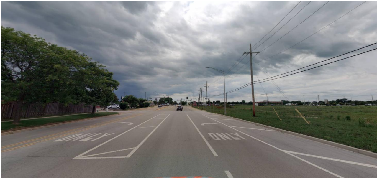
Figure 4: View west down Theodore Street near the east side of the subject site (right) (2026)
