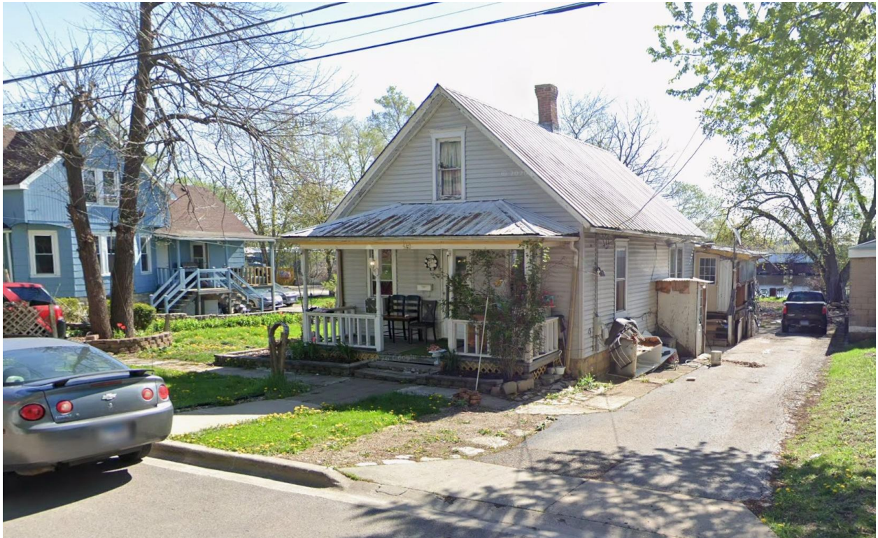
Figure 1: One-story structure at 540 Bluff Street (April 2025)
