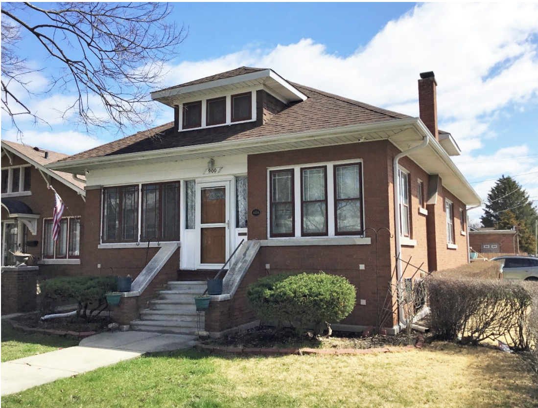
900 N. Raynor, circa March 2022, prior to damage to front façade
