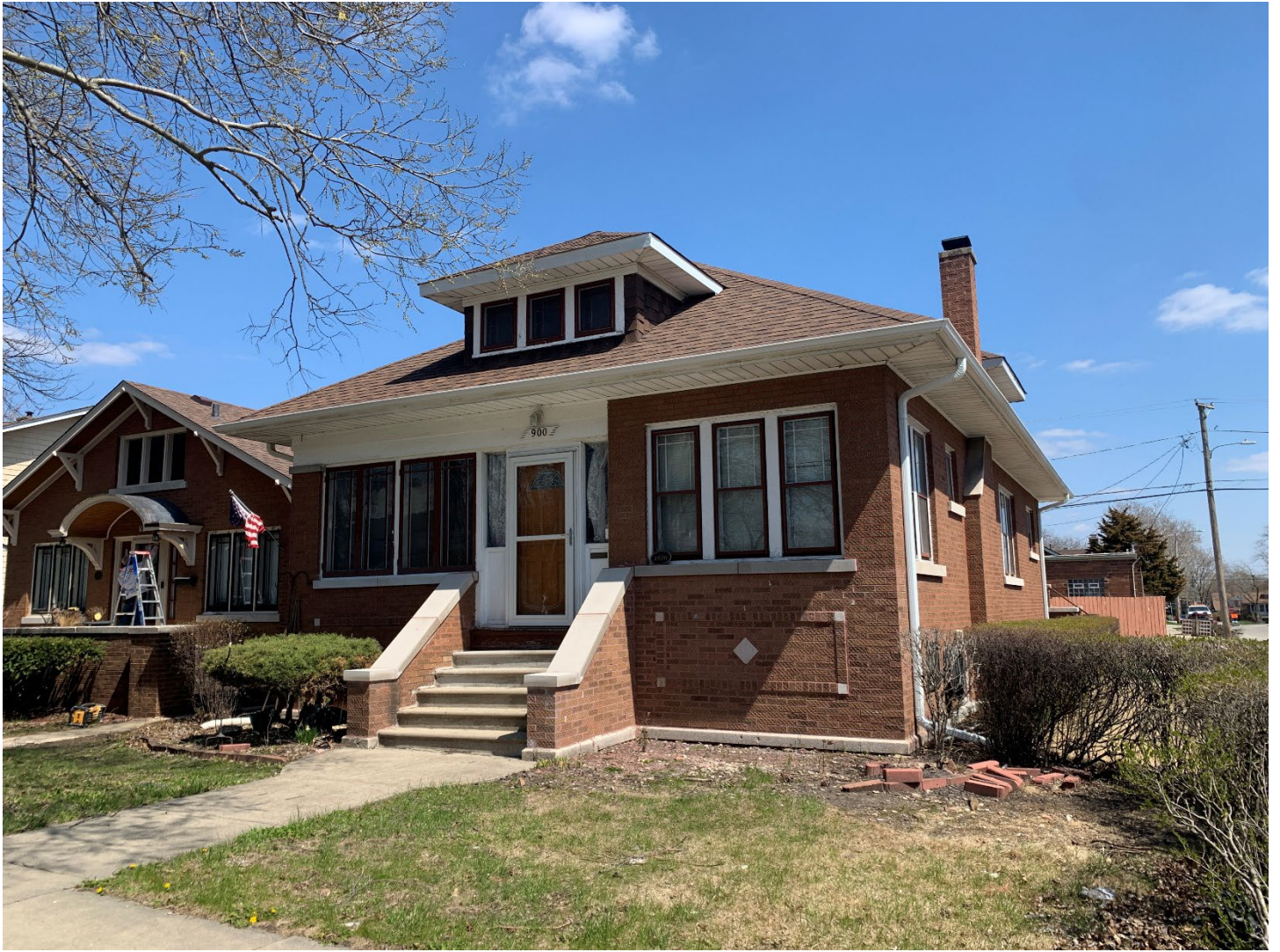
April 2024, shows completed restoration work.
