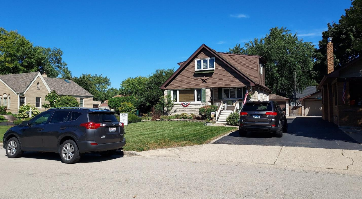
Figure 1: 1307 Briargate Avenue, view north from Briargate Avenue (September 2024)
