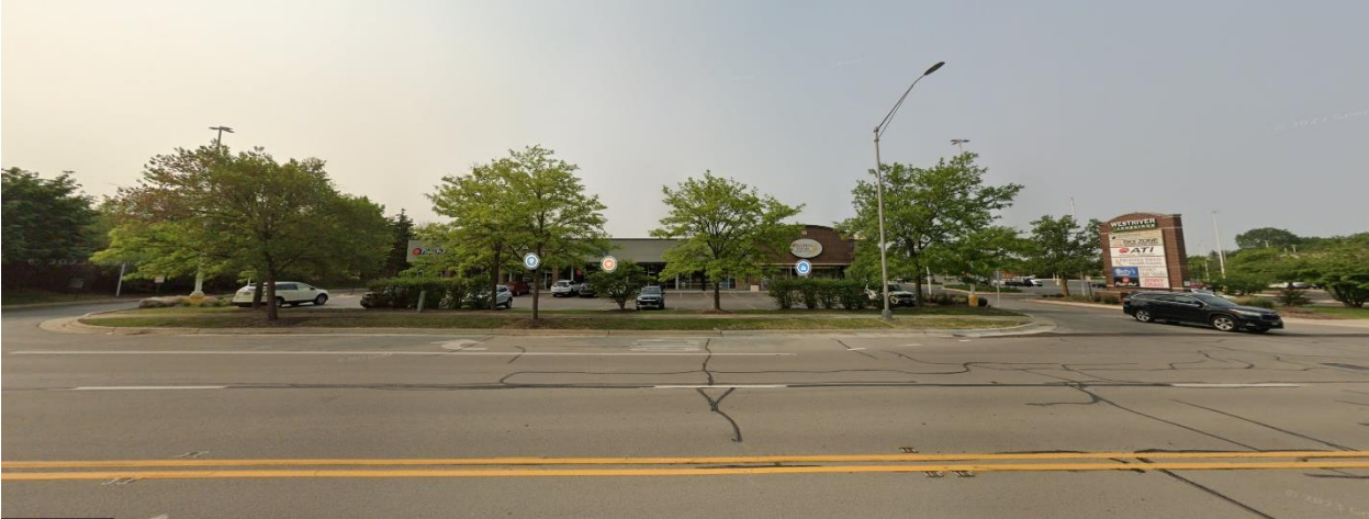
Figure 2: 3038 – 3078 Caton Farm Road, view south from Caton Farm Road (May 2023)
