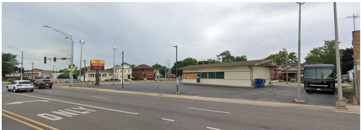
Figure 2: 725 W. Jefferson Street, view northwest from Jefferson Street (August 2024)
