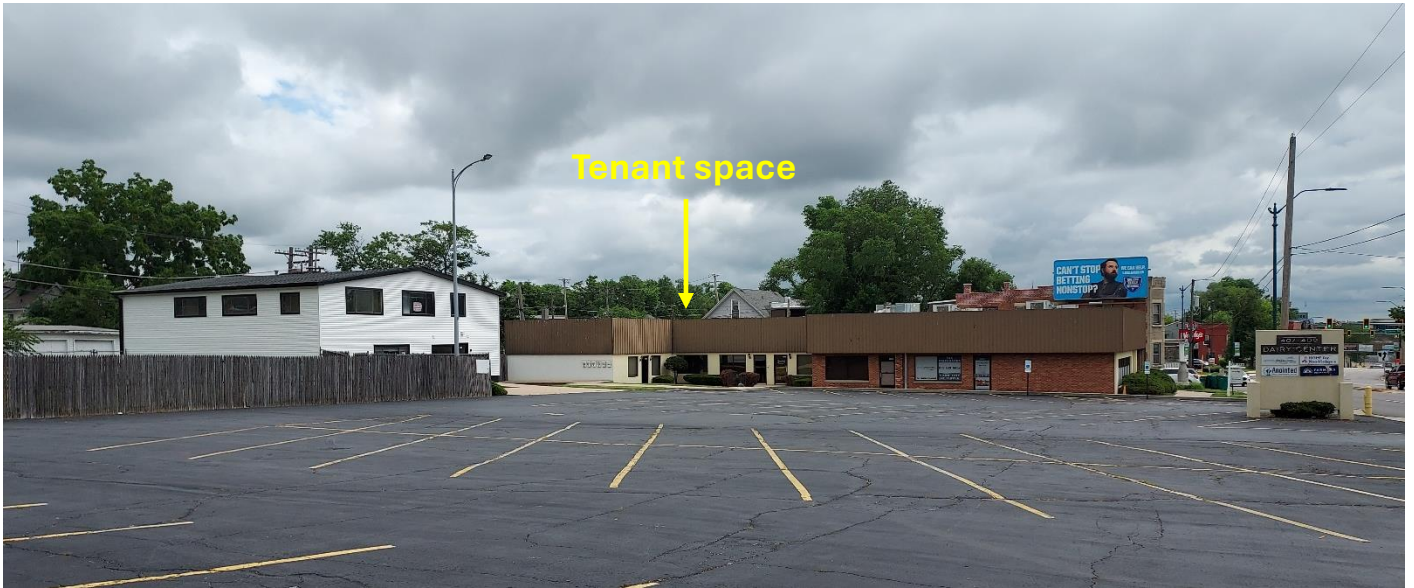
Figure 3: Multi-tenant building at 407 W. Jefferson Street (and 409 W. Jefferson Street on left), view east from subject site parking lot (July 2024)
