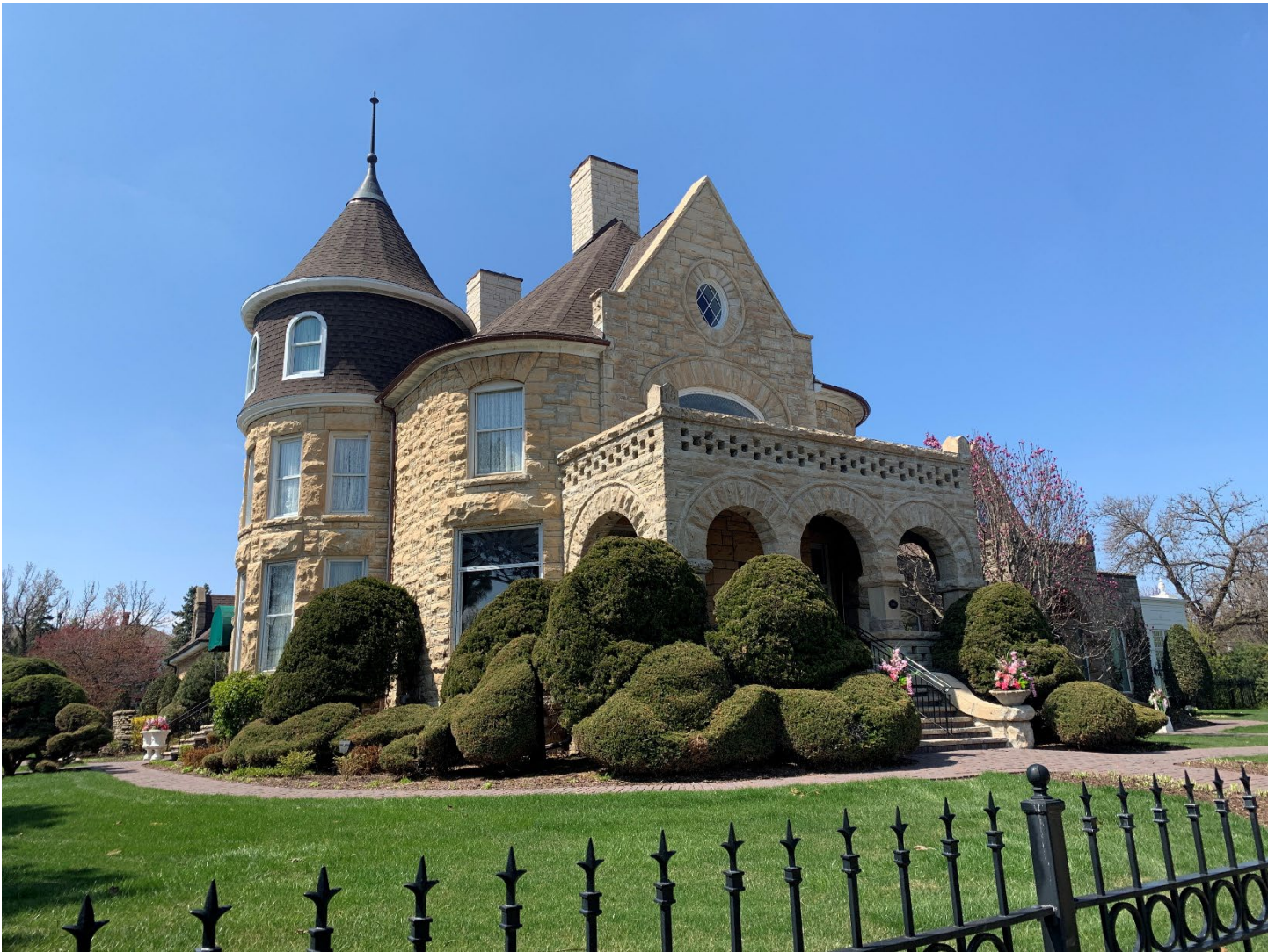
April 2025 after restoration work
