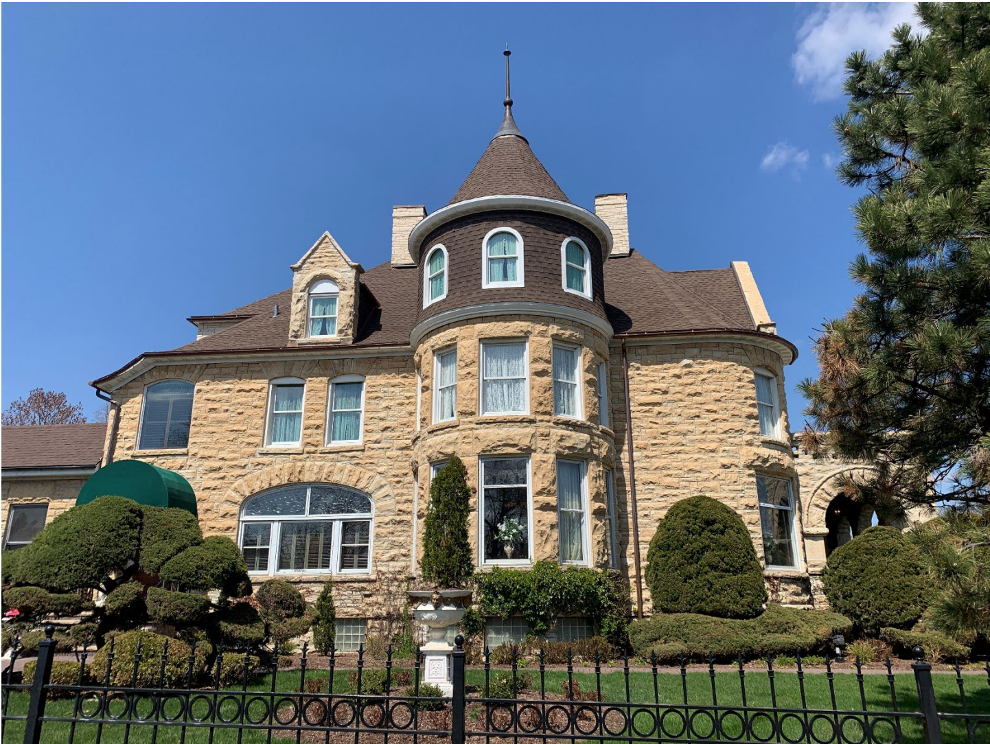
April 2025 after restoration work
