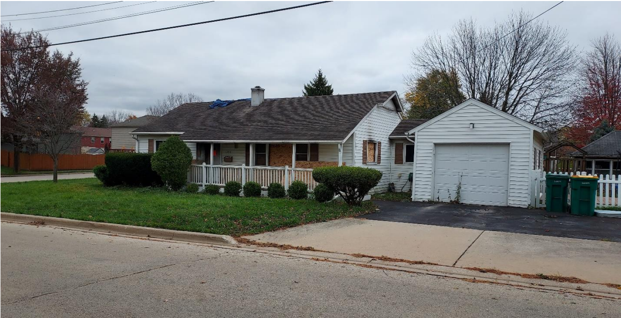
Figure 2: Existing residence at 1150 Norley Avenue, view south from Norley Avenue (November 2024)
