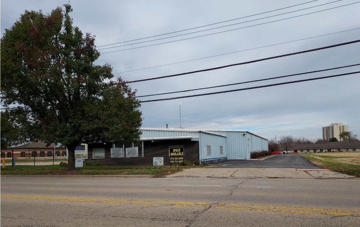
Figure 2: 2705 McDonough Street, view north from McDonough Street (November 2024)
