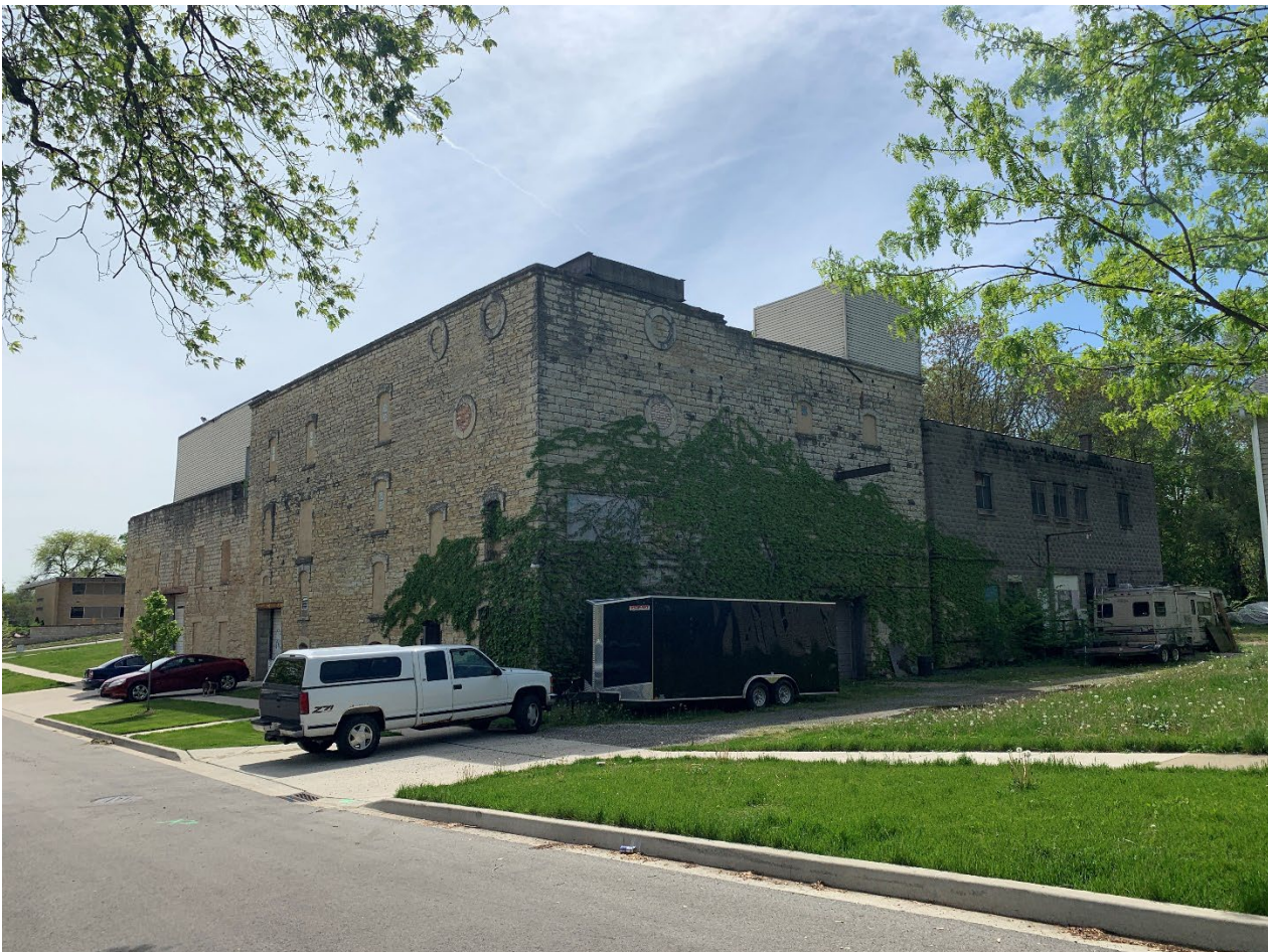
Figure 2: North and east elevations of 515 Summit Street
