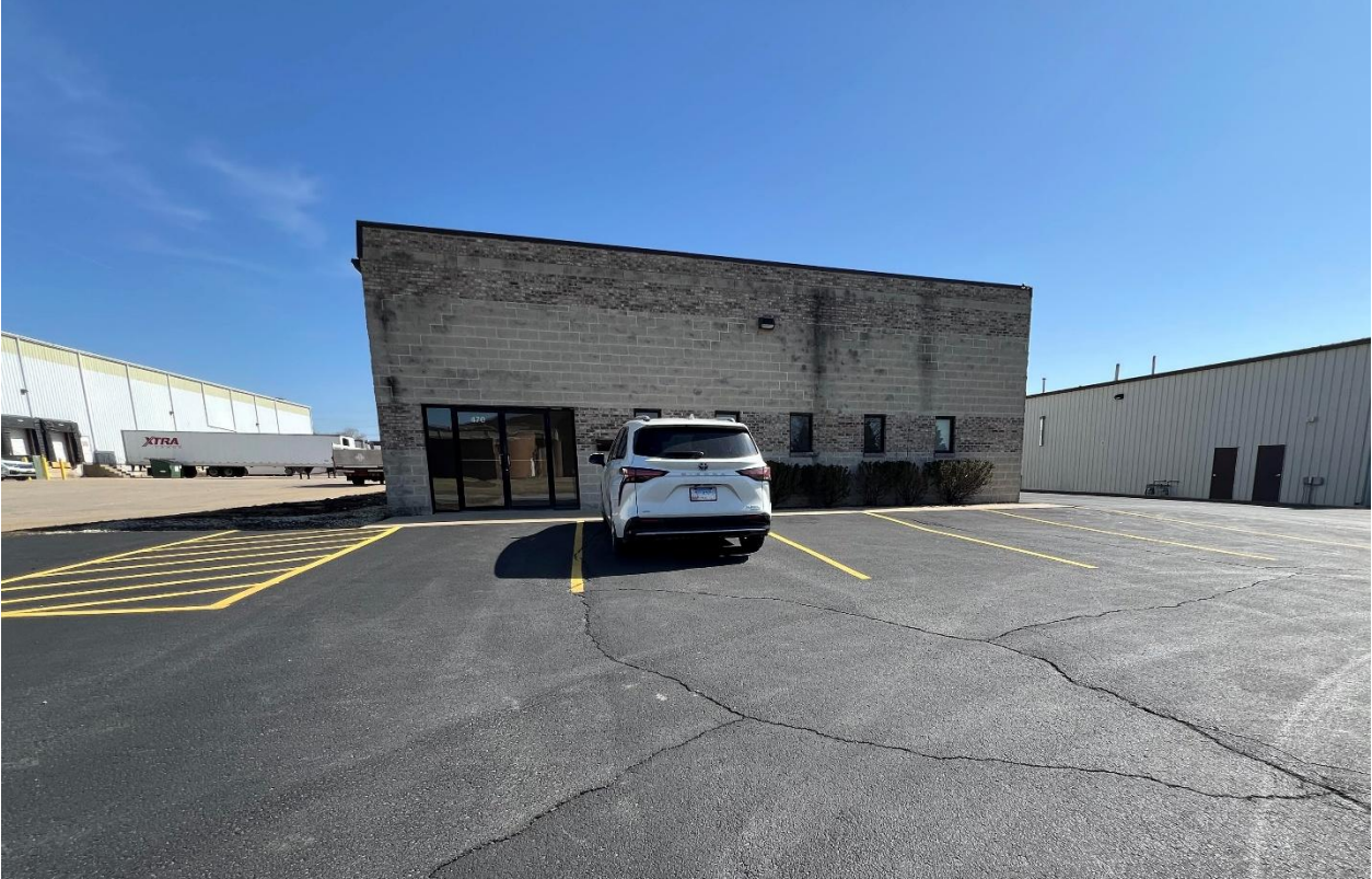
Figure 3: 470 S. Hammes Avenue, view east from Hammes Avenue (March 2025)
