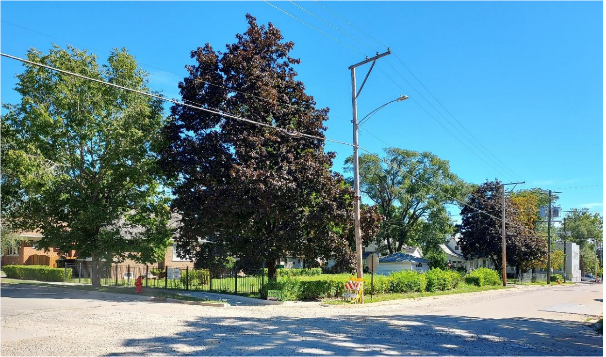
Figure 2: 1000 N. Center Street, view northeast from intersection of Center Street and Moran Street (September 2024)
