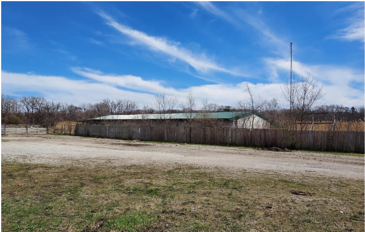
Figure 6: Former Joliet Beach Club concession stand located on annexation parcel – future storm detention area
