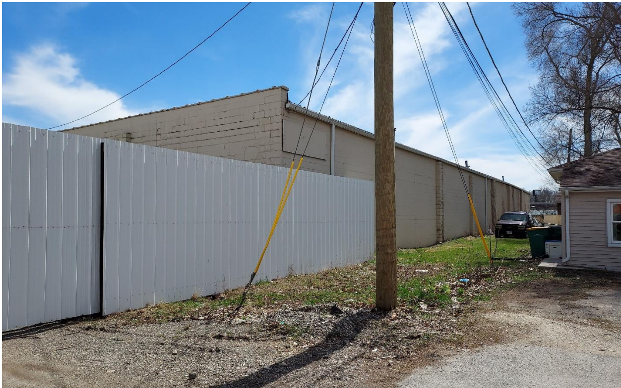
Figure 8: West side of existing concrete block building, view south from Fourth Avenue
